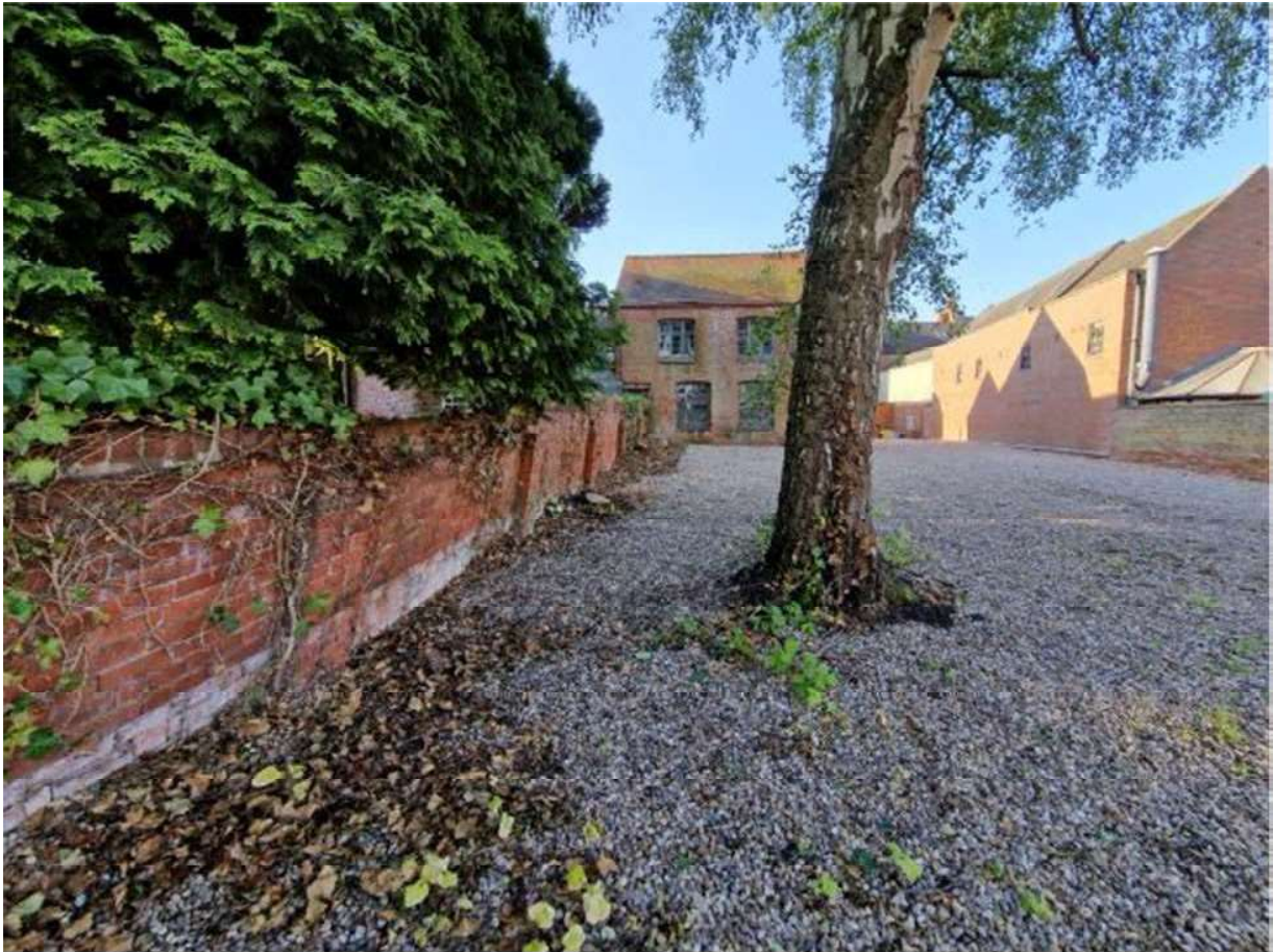
Tree is very close to the wall causing it to become unstable.
