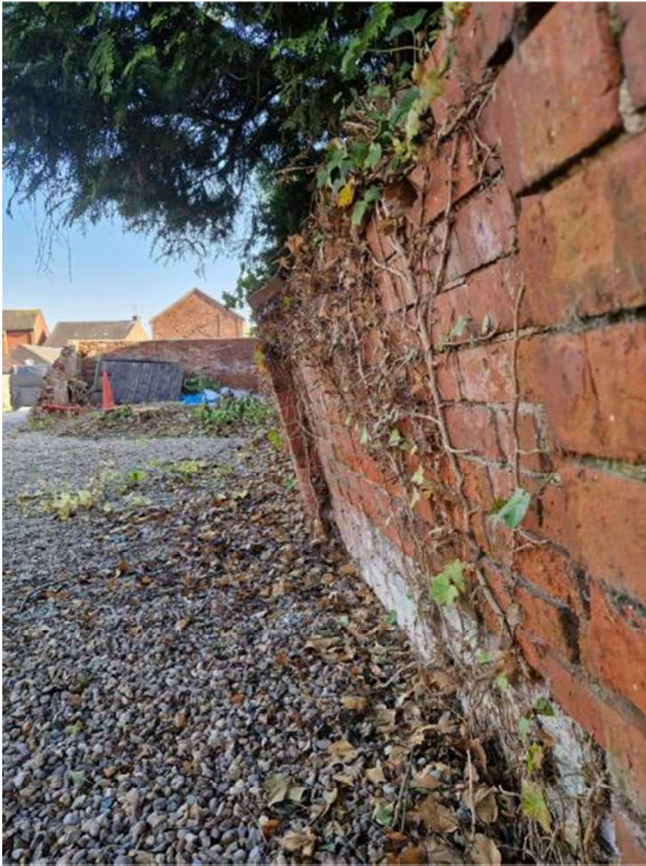
The wall is leaning at such an angle that it is unstable.
